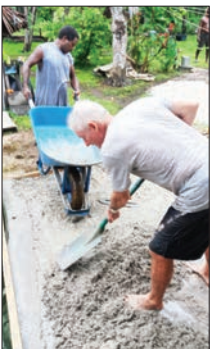
Peter laying the cement slab
