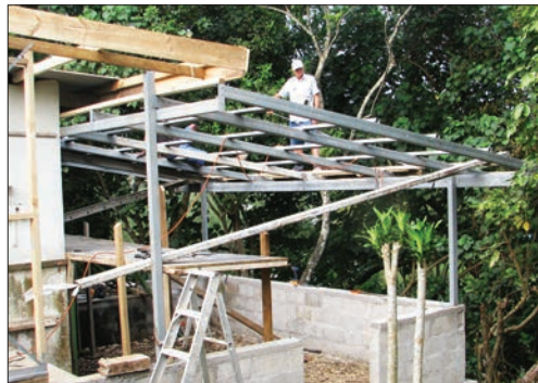
Denis working on Loui's house
