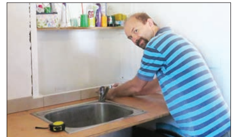
Miklos placing tiles on the splash-back
