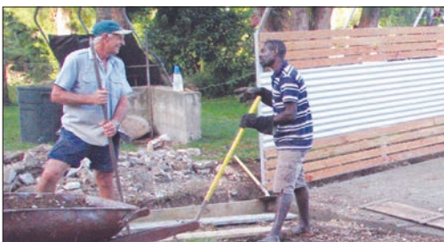
Denis and Loui working on the driveway
